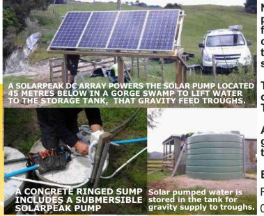
Need water pumped on that farm from a creek or bog up to a header storage tank?
