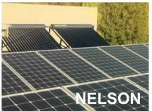
An executive multi leveled home combines 40 tubes retrofitted to a 350 litre external cylinder together with a 6 kW photoelectric system grid tied giving the owners a very sophisticated energy system
