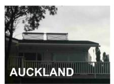
This 4 bedroom home combines 40 tubes with a solar ready superheat twin element cylinder.Again a dishwasher and washing machine gets it's hot water from this system.
