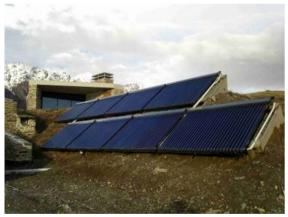
**This celebrity** home combines 240 tubes with a solar ready combination 1000 litre tanks and a heatpump for underfloor domestic heating, A floor heated pool system uses the extra summer energy. A reflection pool has floor pipes to stop it freezing in winter.
